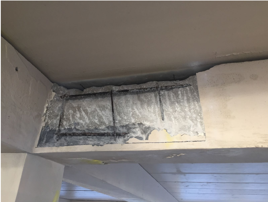
Picture 1: In-progress demolition
