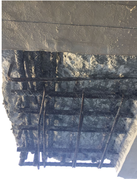
Picture 3: Repair requiring stirrup supplementation
