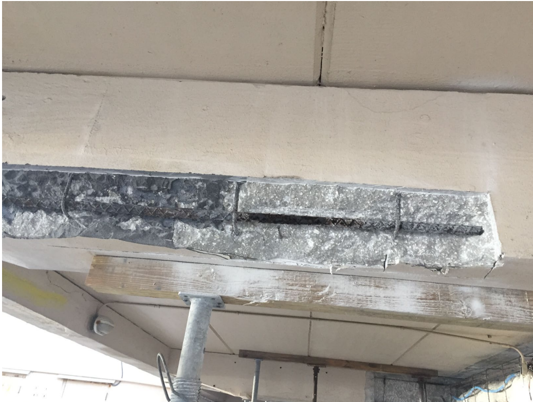
Picture 2: In-progress demolition
